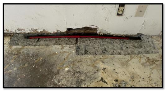
All 6 new full-length cables installed at north and south ends of 3<sup>rd</sup> floor slab at makai side of the building
